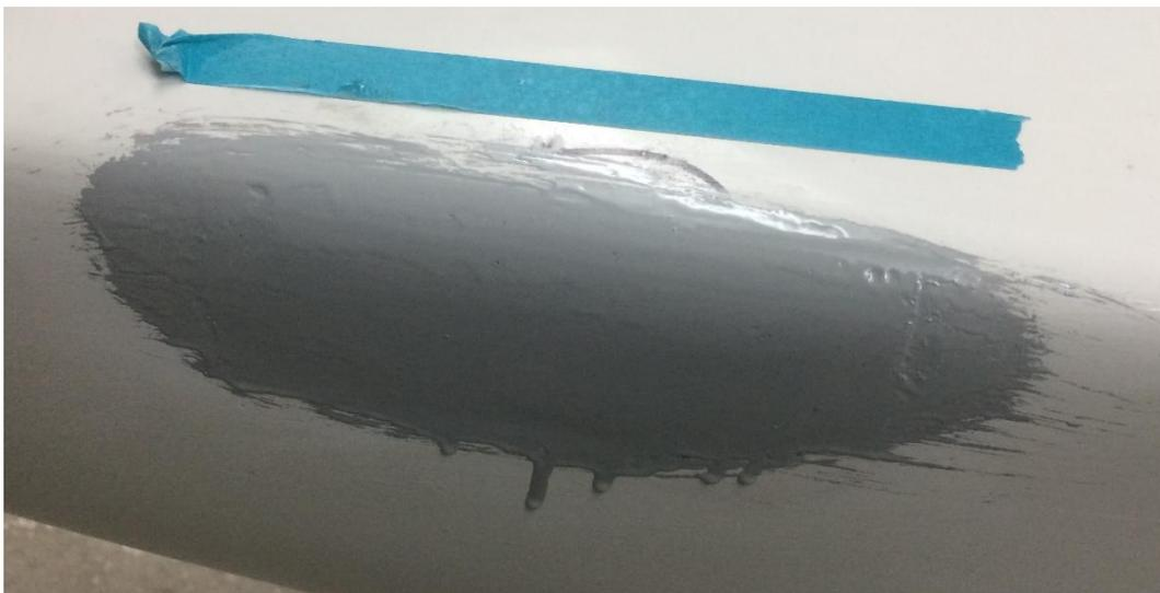
3. When the primer is dry, use a plastic putty card to fill where needed with polyester filler, do not overfill the area. It is much better to fill several times and sand again with 100 grit and sanding block lightly between fills
