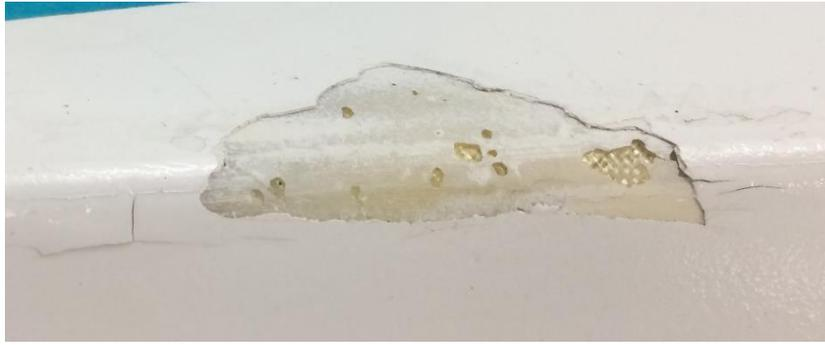
3. Grind all the broken areas away so there is only good unbroken fibreglass left around the hole, then taper the edge for about 50mm back into unaffected hull to create a scarf.
